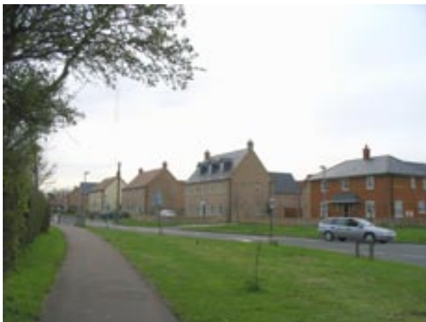
West end of Church Street, looking towards the recent housing development
