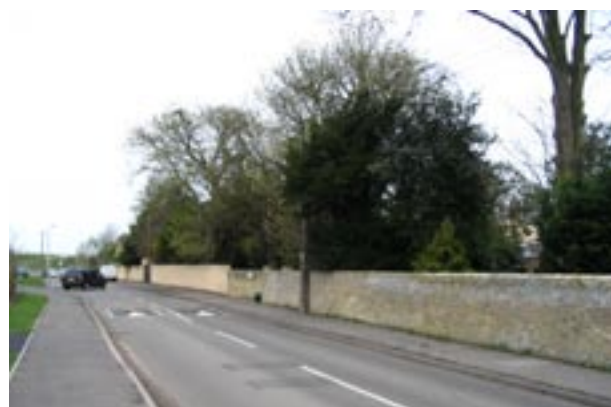
View west along Church Street
