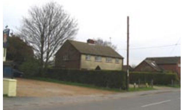
C20 semis & public house parking area
