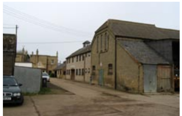
C19 barn & outbuildings at Teversham Hall Farm
